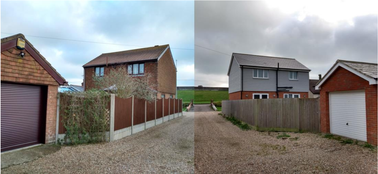
Photo 4: Rear of 1 and 2 Willop Close
